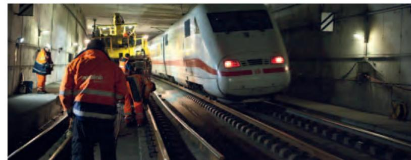
Rail replacement in a tunnel – traffic flow continues uninterrupted on the adjacent track
