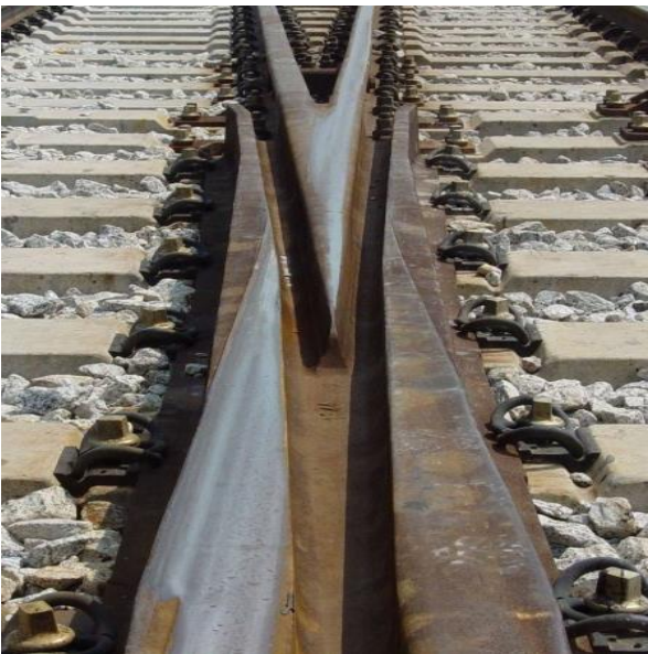
Crossing with Vossloh W30 HH fastening system ➔ reduction of maintenance costs by permanent elastic tensioning of the rail with tension clamps.
