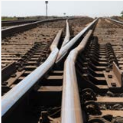
Crossing with Vossloh W30 HH fastening system
